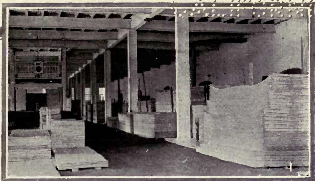
1, 2 and 3.— Creosoted wood block floors in the Follansbee Tin Plate Co., Follansbee, W. Va. These floors must withstand the wear and tear of heavy trucking
