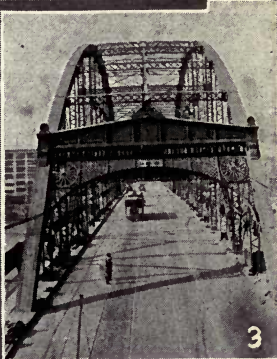
1.—A bridge floor of creosoted wood blocks
