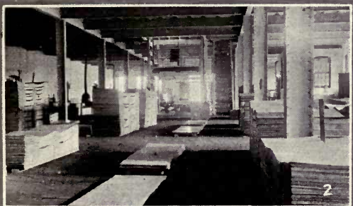
1, 2 and 3.— Creosoted wood block floors in the Follansbee Tin Plate Co., Follansbee, W. Va. These floors must withstand the wear and tear of heavy trucking
