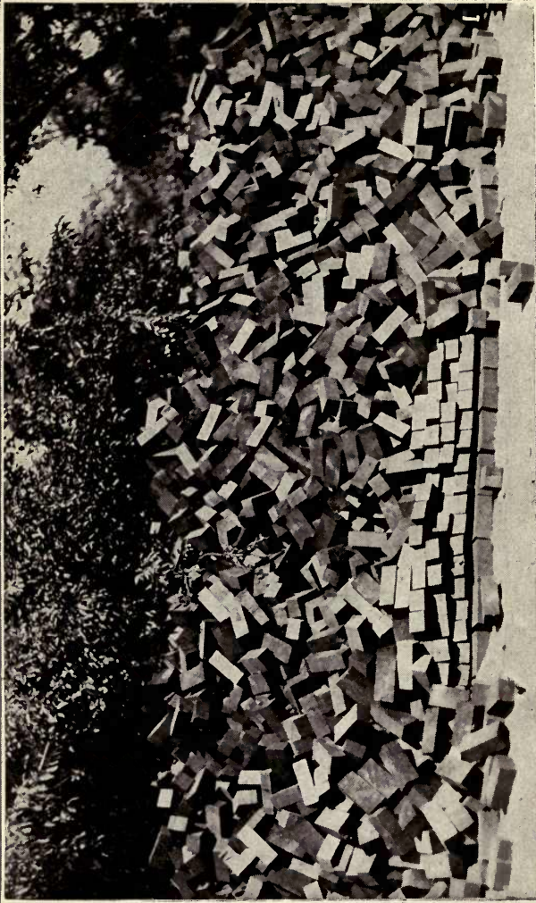
Creosoted wood blocks. When made by Creolignum standards they are absolutely uniform in size and shape and preserved against decay to last for the full life allowed by the traffic which eventually wears them out
