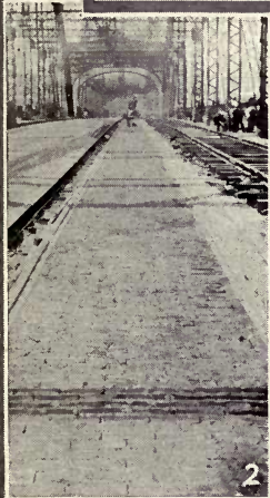
1.—A bridge floor of creosoted wood blocks
