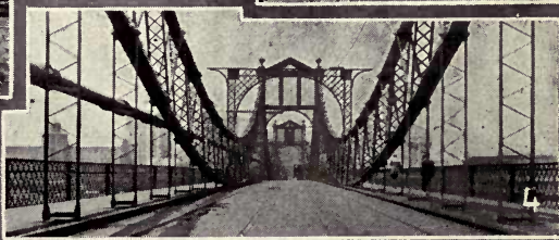
3 and 4.—Bridges where the creosoted wood blocks of the floor give promise of longer life and require less care and attention than the structural steel of the bridge itself
